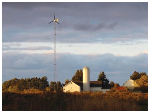
Figure 1. A rural residence with a Bergey Excel 10 kW turbine with a 23-ft rotor located in Charlotte, Vermont.
